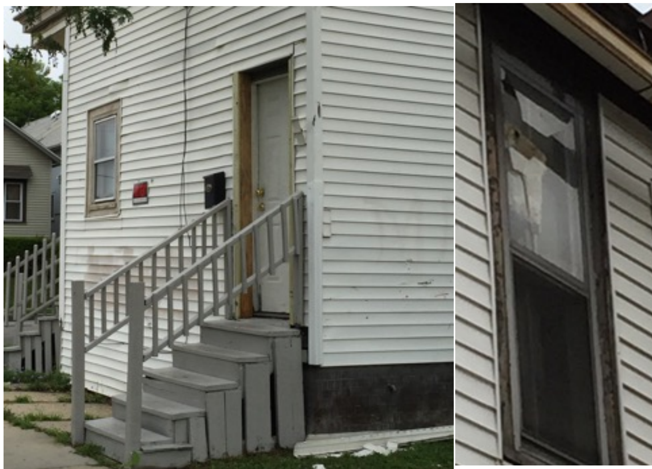
1532 W Scott - Immediate to the west Siding,rails, paint, broken windows.
