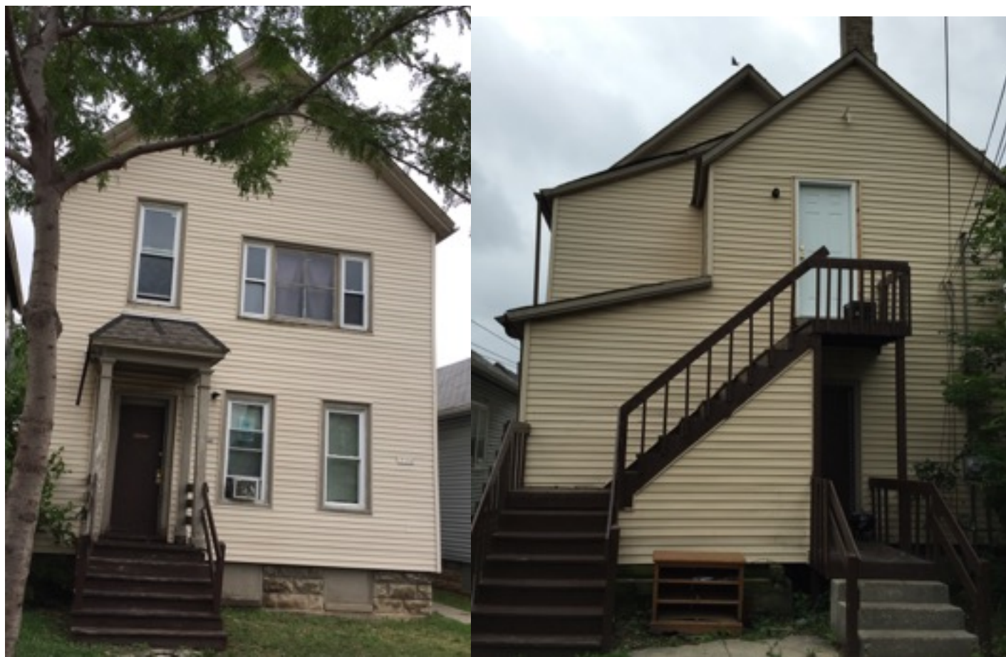
1532 W Scott - Immediate to the west Siding,rails, paint, broken windows.
