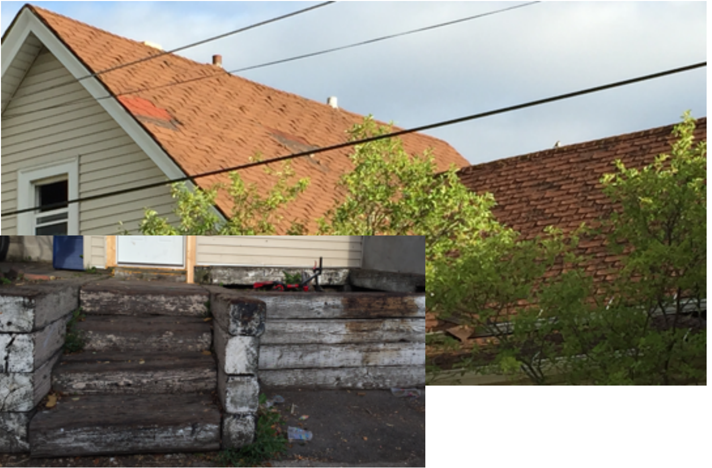
1440 S 10th Roof/ retaining wall/steps
