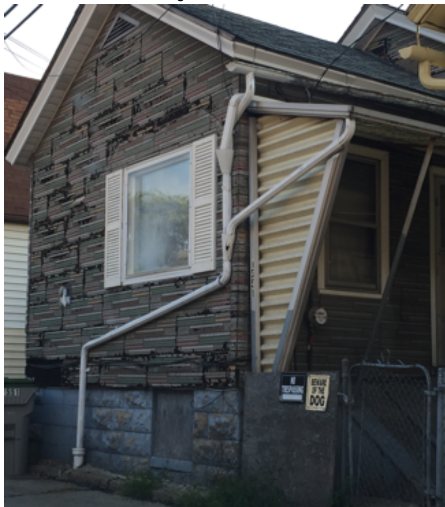
1551 S 10th. Siding/Paint/Gutters/Fence
