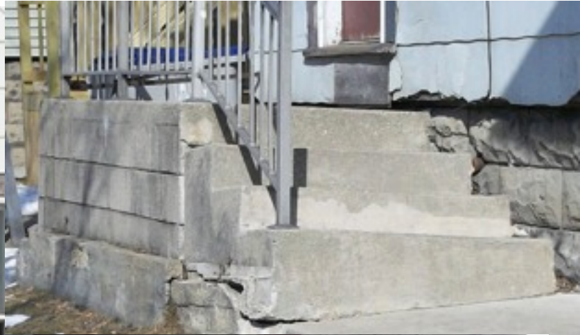
1424 S 6th Adjoining North Missing siding, needs paint, defective front steps needs paint, siding, front step is defective, sidewalk is defective.
