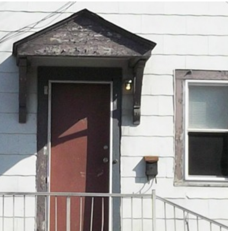
1424 S 6th Adjoining North Missing siding, needs paint, defective front steps needs paint, siding, front step is defective, sidewalk is defective.
